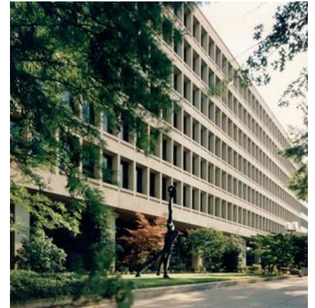
Federal Reserve Annex
